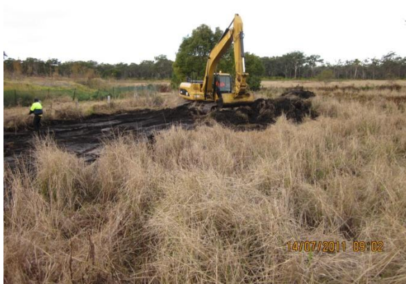
Stripping of vegetation and topsoil from proposed lot fill area
