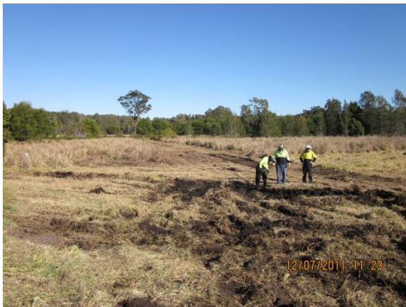
Site prior to stripping and filling. Route of east-west trending access road across site roughly delineated by existing track
