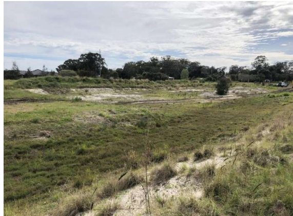
Looking north showing stockpiles of dredged sand in the central part of the site.
