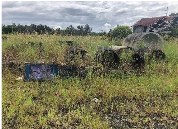
Looking west showing stored concrete bollards and pipes and an old shed in the background located on the western side of the access road.
