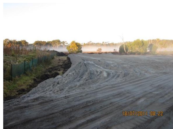
Sand fill placed over lot fill area following stripping of topsoil
