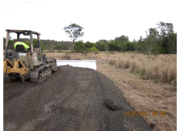
Access road fill comprising imported crushed rock material, placed over geofabric placed directly over the existing surface.
